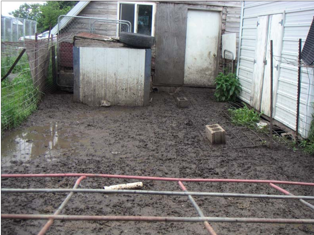
Mud and Standing Water; Rusty Metal and Bent Wire; Broken Shelter; Tire Covering Torn Roof of Shelter; Fencing Material on Ground
